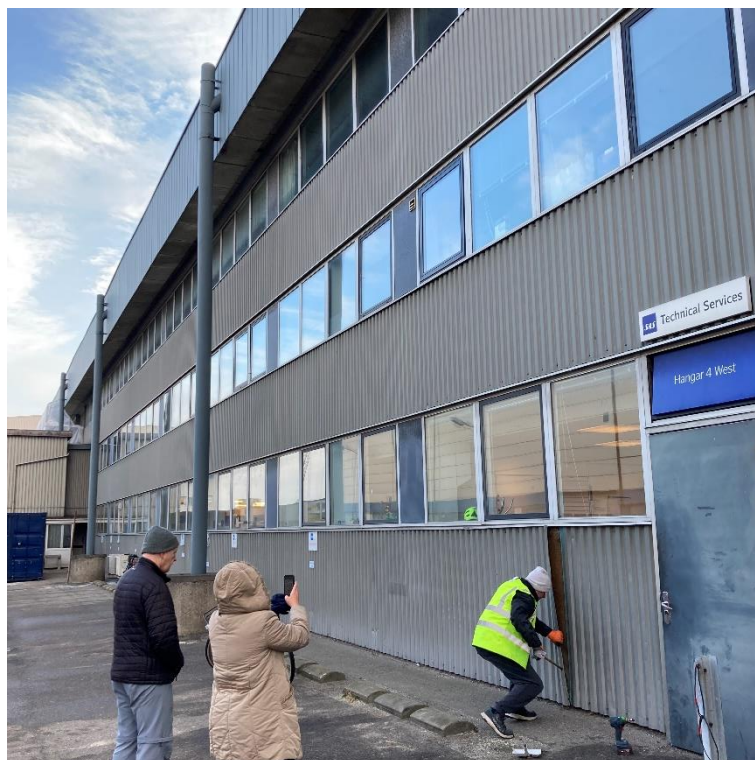
Figure 1. Photo of CPH Hangar 4. Insulation samples were covered by trapezoidal metal wall panels.
