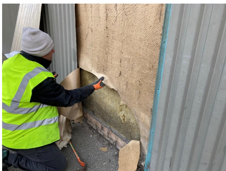
Figure 2. Insulation slabs behind trapezoidal metal wall panels and cardboard wind-stop.
