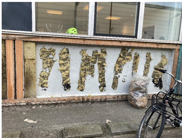
Figure 3. Insulation slabs were glued to the wall.
