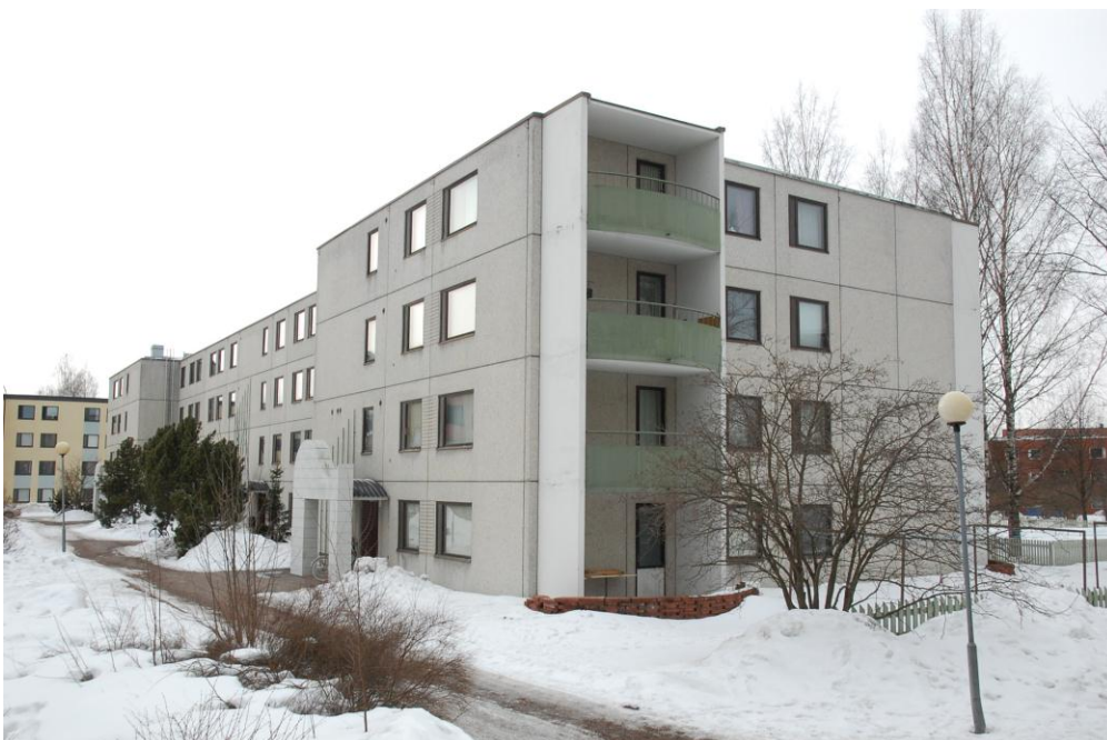
Fig. 1 The multi-storey house in Saturnuksenkatu 2, Riihimäki is retrofitted to meet the Finnish passive house requirement, i.e. the heating energy demand after the renovation is max. 25 kWh/m 2 a. Photo: Jari Kiuru.
