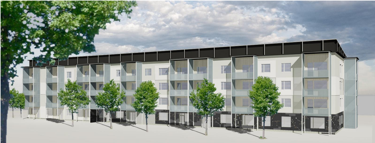
Fig. 5 The new façade materials are plaster rendering, cement fibre board (day-care centre) and wood cladding (balconies). The 3-dimensional surface of the plaster rendered facade and the variation of colour show the division of apartments behind the façade. The target of the architectural design was to upgrade the facades, but still maintain a connection to the original character of the building. Image: Kimmo Lylykangas Architects.
